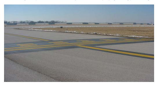
When ATCT is in operation, the controller may ask you to hold short of the runway. In this case, you must stop before the hold line and proceed only after you are cleared to do so by the controller, and you have checked for traffic. During the periods that ATCT is closed, you should stop and check for traffic and cross the hold line only after ensuring that no aircraft is using the runway for landing, takeoff, or taxi. When exiting the runway, do not stop until you have cleared the hold line.
